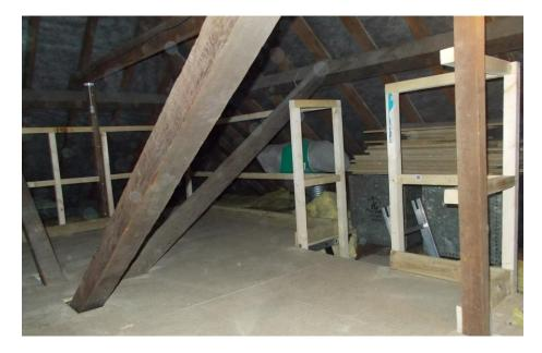
LoftZone has developed a raised decking for lofts, which protects insulation from compression, whilst allowing safe access to workers. Recent research by the National Physical Laboratory and Carbon Trust has shown that loft insulation is compressed in most UK houses, and that this reduces its effectiveness by 50-60%. The LoftZone raised decking won Best New Invention 2013 at the Ideal Home Show in London.
