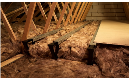
Storage deck in a house
