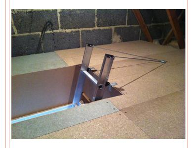
(3) You can fix a ladder on to a joist and stow it away from the deck.
